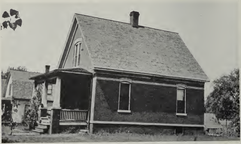
FIG. 44.—Houses in northwest Springfield for which claims were paid by a mining company for damages caused by mining a coal 5 feet 9 inches thick at a depth of about 200 feet.
